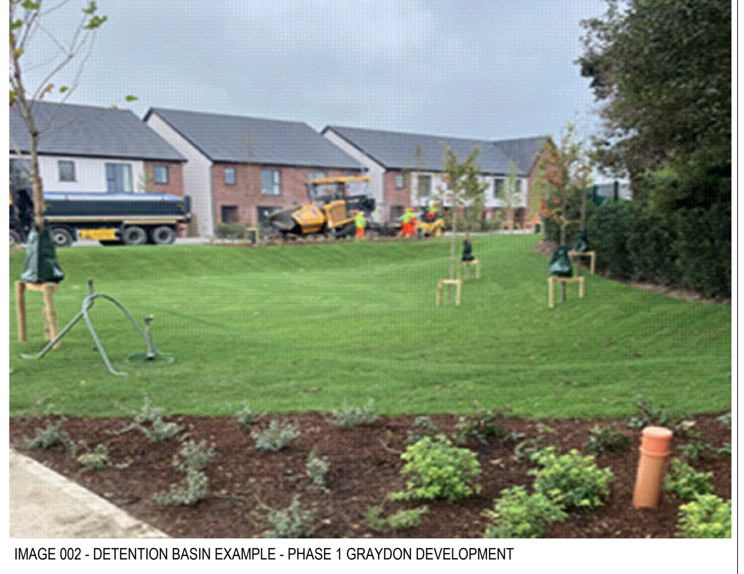
IMAGE 002 - DETENTION BASIN EXAMPLE - PHASE 1 GRAYDON DEVELOPMENT
